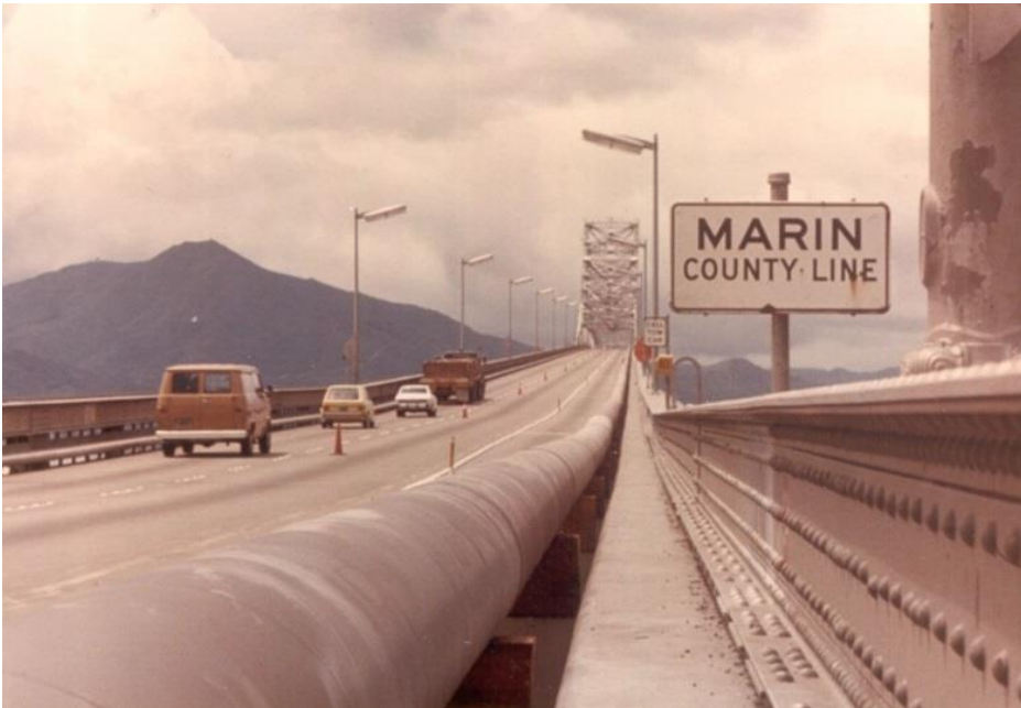
Richmond San Rafael Bridge Water Pipeline 1973 (Courtesy of MMWD)
