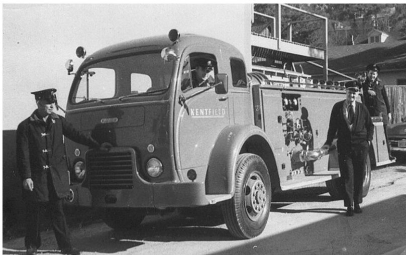
Keeping firefighting equipment up to date has been a priority at the Kentfield firehouse. The 1960 Van Pelt/White truck. (Kentfield Fire District Collection)
