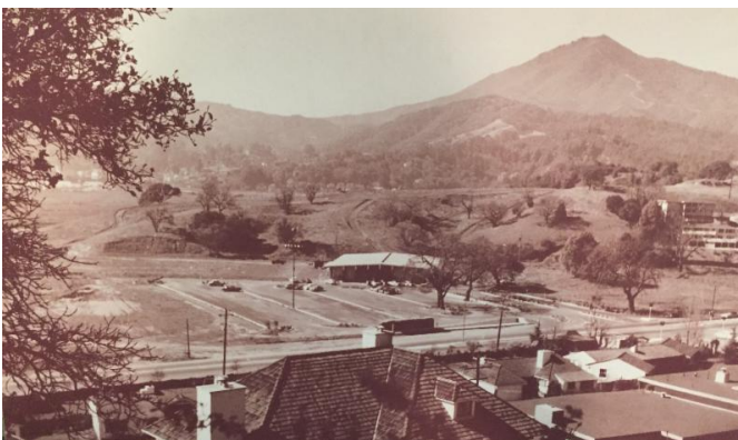
Building Bon Air Center 1950's (Greenbrae Management Inc)
