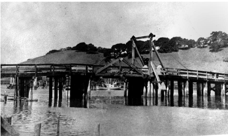
The one-lane drawbridge was part of the "Tiburon Boulevard" road constructed across the marshes to San Rafael around 1900. (Courtesy of the Larkspur Heritage Preservation Board)
